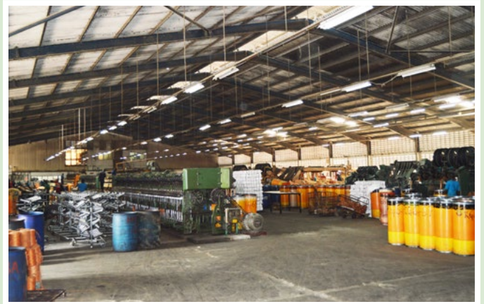
21st Century Holdings factory premises
